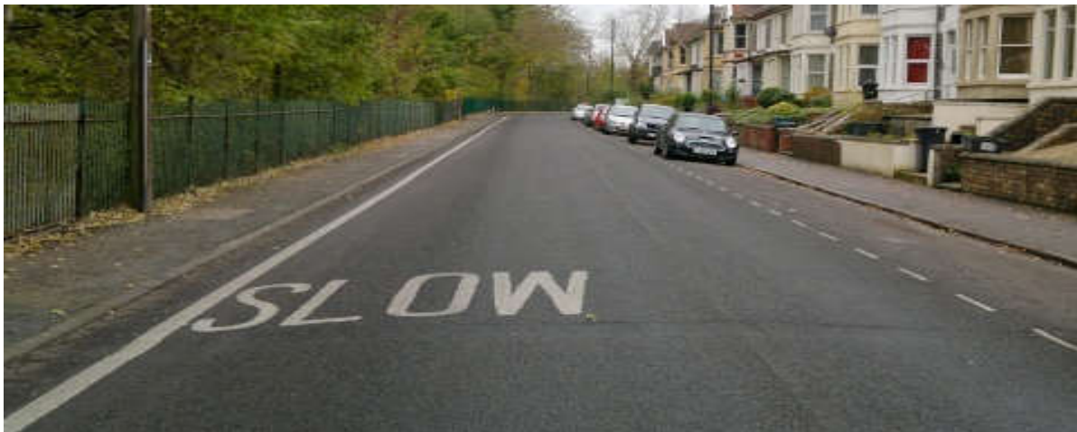
Figure 8 - Example of edge of carriageway marking
