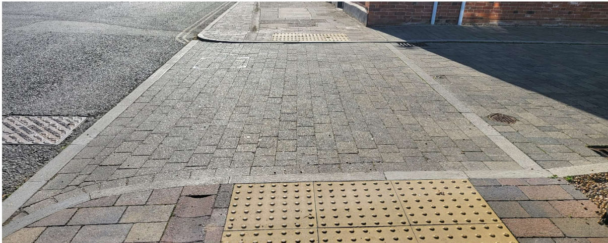
Figure 16 – Example of uncontrolled crossing without central island
