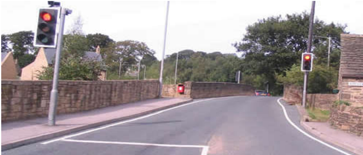
Figure 24 – Example of a traffic signal shuttle system in operation on a bridge
