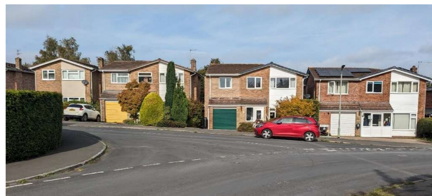
Figure 4.3 Poor quality play area (top), missing footway (middle-left), poor quality and inaccessible bus stop (middle-right), and excessively wide junction mouth (bottom),
